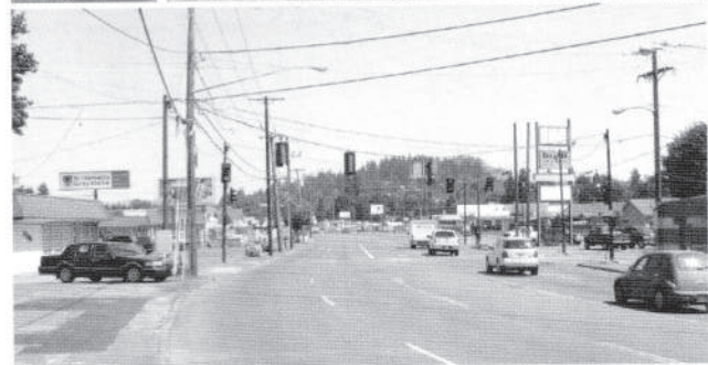
Franklin Boulevard, which runs right through Glenwood, will get a major multimodal overhaul: dedicated transit service, enhanced bike and pedestrian facilities, and roundabouts.
