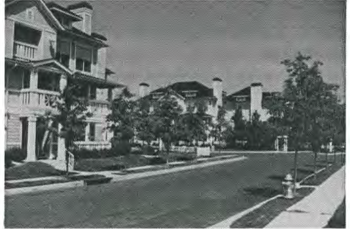
Eight-plex apartments which treat internal drives as public streets, Harbortown, Memphis, Tennessee
