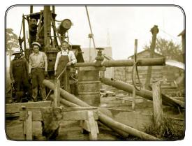
Tapping into the groundwater, as a means of supplementing decreasing supplies, ca 1932.
